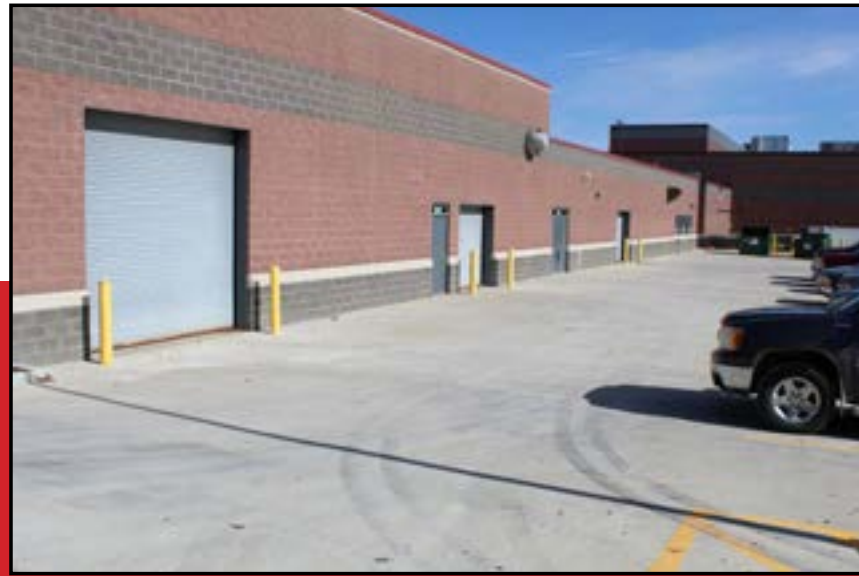
Concrete Delivery Area
